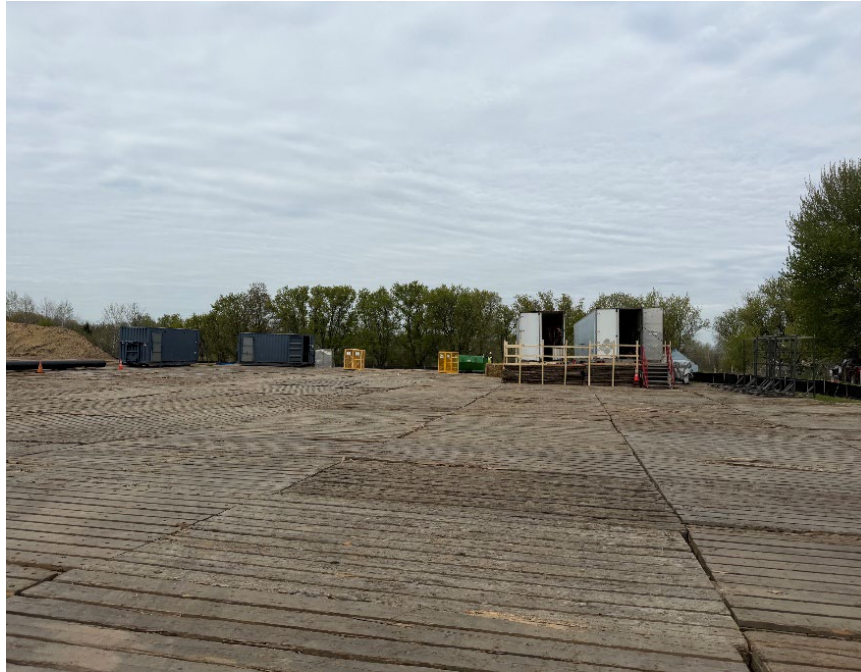
Facing west near MP 3.4, staging area topsoiled and matted
